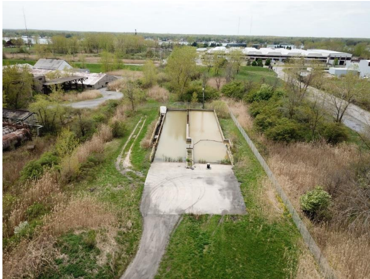
Photograph No. 2 Settling Ponds (View Looking West) Before Aeration Testing May 2020
